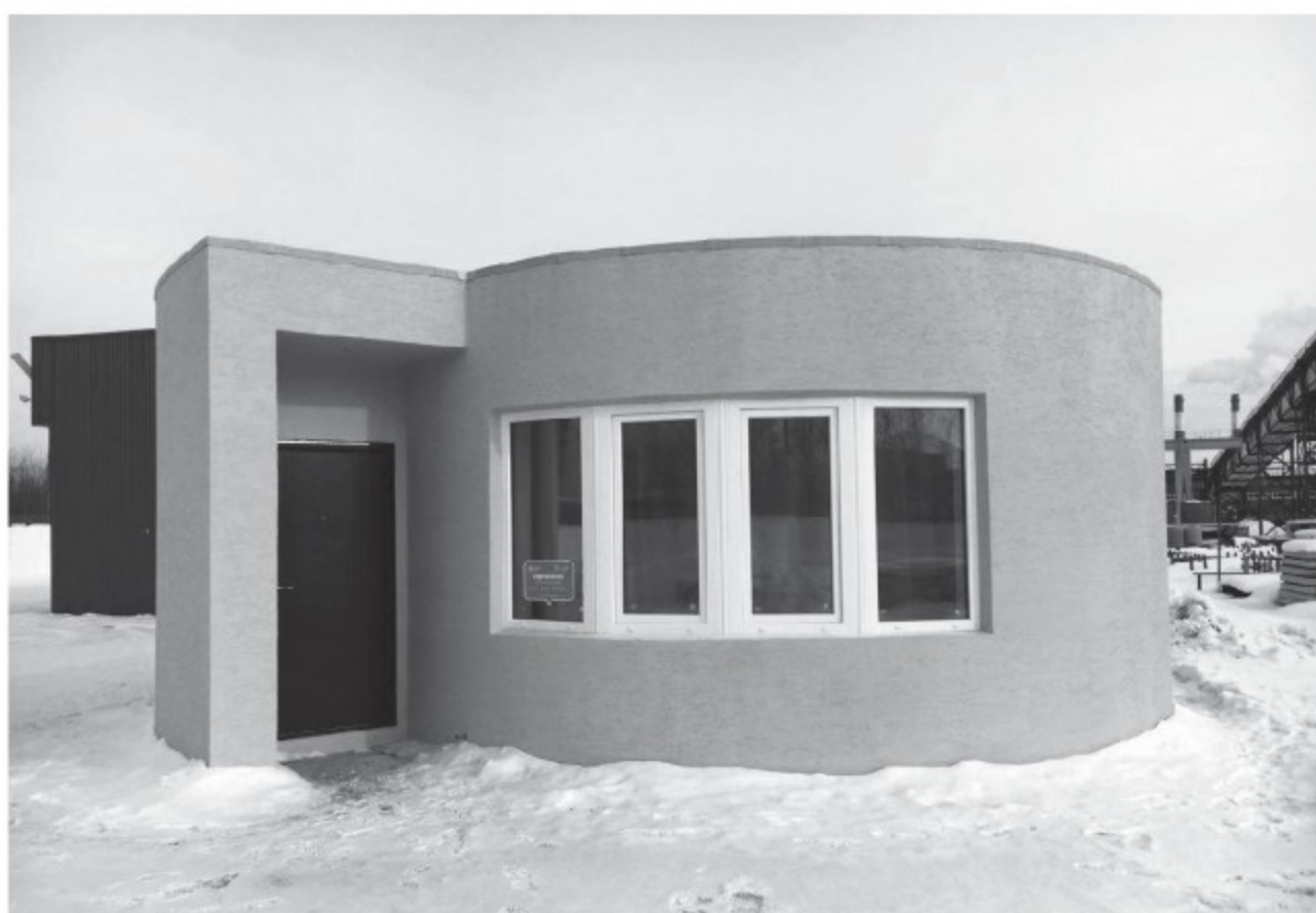
▲ The 3D-printed house in Russia
